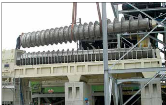
Figure 7. Babbini press installation
