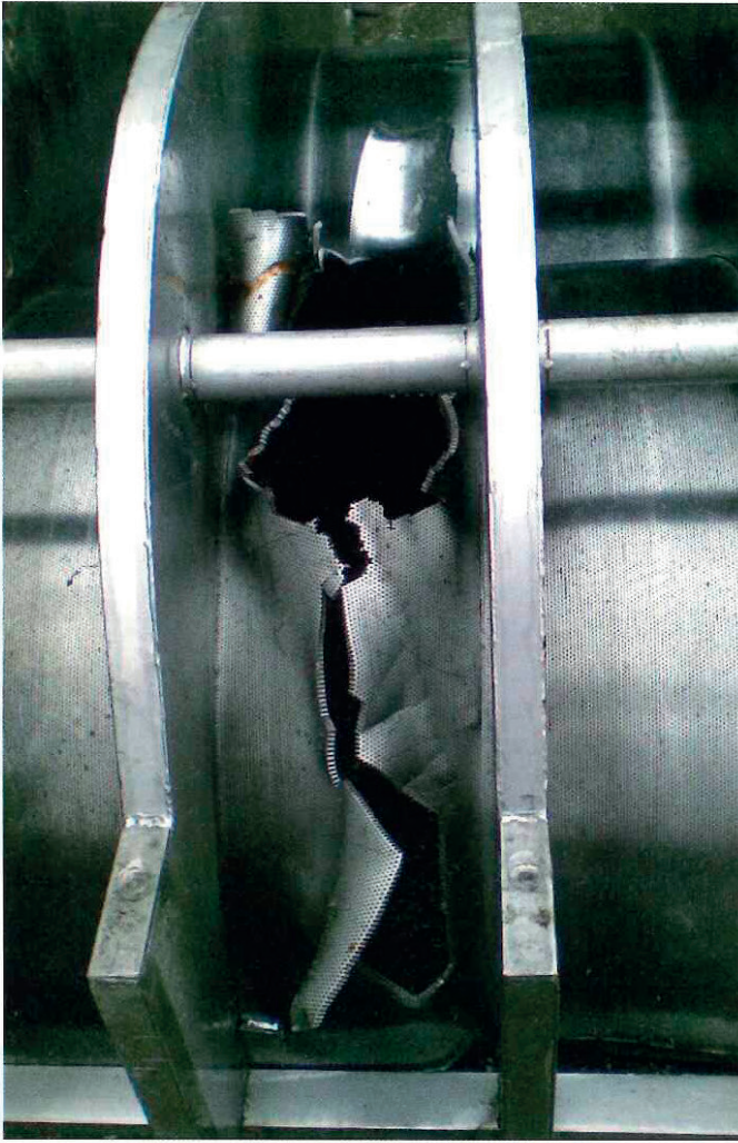
Fig. 1: Damage due to the entrance of a foreign object
